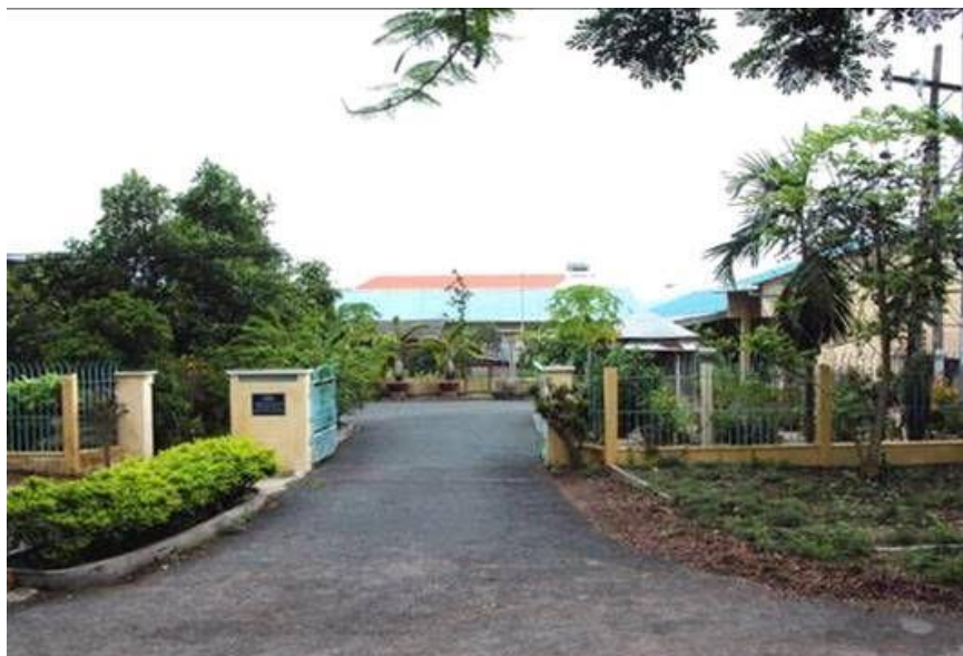
Figure 10 Old building of the Biotechnology Research and Development Institute
